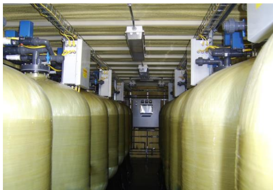
Figure 2- Advanced staggered bed system utilizing fixed bed design
