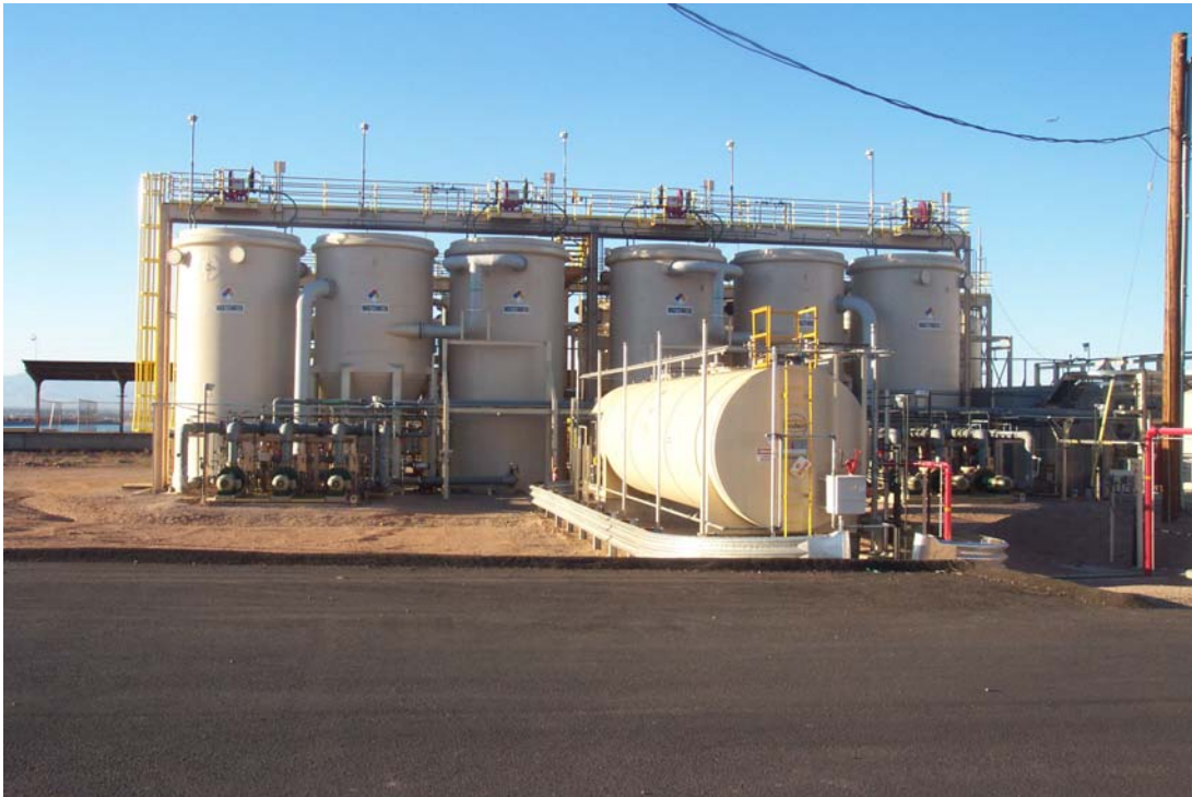
Figure 1. First stage sand FBRs and electron donor storage.
