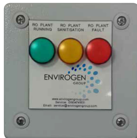
Remote wall-mounted alarm indicator
