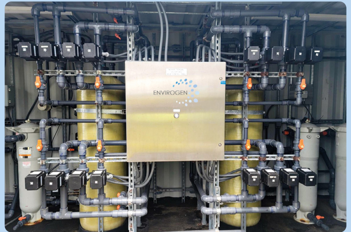
Envirogen's SimPACK (Left) and MinX (Right) regenerable IX systems, delivered as a containerized solution.
